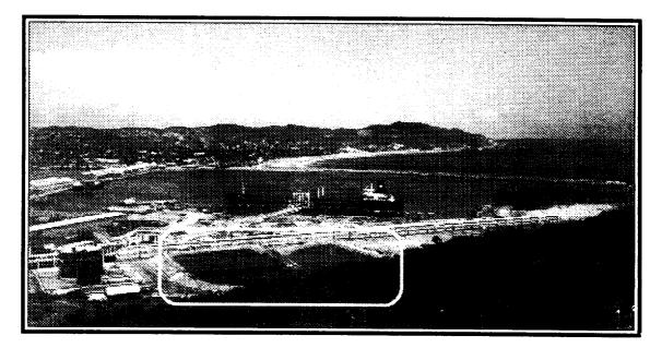
Fig. 3. Refinery port with lagoon for oillwater separation
