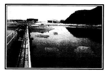
Fig. 4. Lust step in oillwater separation lagoon. Note patches of oil on the water.
