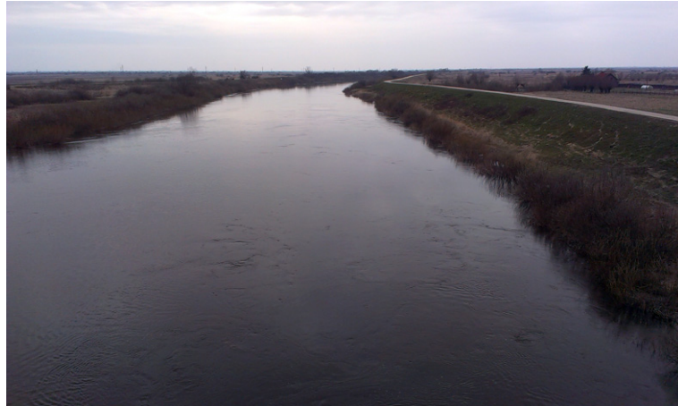
Figure 2.167 – Matrosov Canal Bed Reach, in downstream direction (Photo: Pilipchuk, 03.04.2014)
