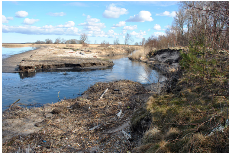
Figure 2.158– Kaliningrad Canal Bed Reach, in upstream direction (Photo: Domnin, 01.04.2014)
