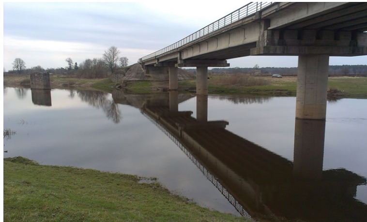
Figure 2.153 – Sheshupe River Bed Reach, in downstream direction (Photo: Pilipchuk, 03.04.2014)
