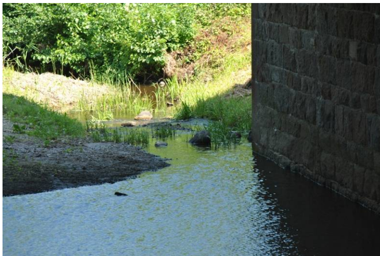
Figure 2.20 – The River Bajdukovka Bed Reach, in downstream direction (Photo: Domnin, 04.07.2013)
